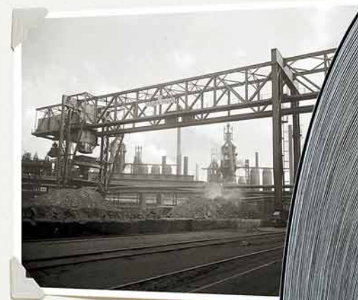
Coal loading with new loading bridge
